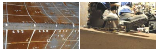
Figure 6 Crack in the centre of the V-corner (left), view at floor section with broken supports and lifted feet (right)
